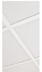
Suspended Ceiling Grid
